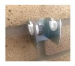
Wall Brackets — Offer up the radiator in the desired position, mark the bracket positions and fixing holes. The radiator should be placed a minimum of 10cm from the floor. Using the appropriate drill and fixings attach the brackets to the wall. After installing the plastic inserts into the hook part of the bracket the radiator can then be hung from the brackets.
